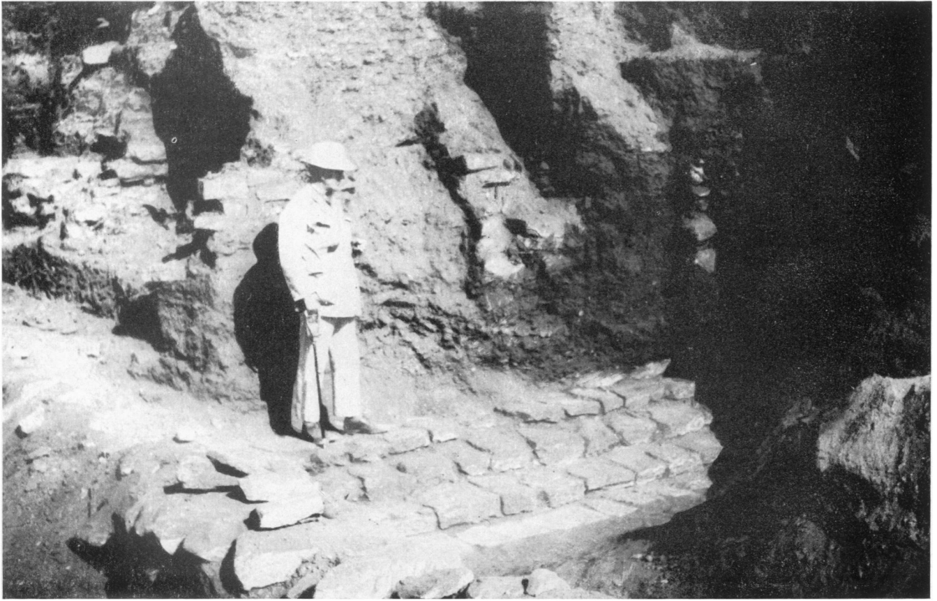
1. The East Stairway
